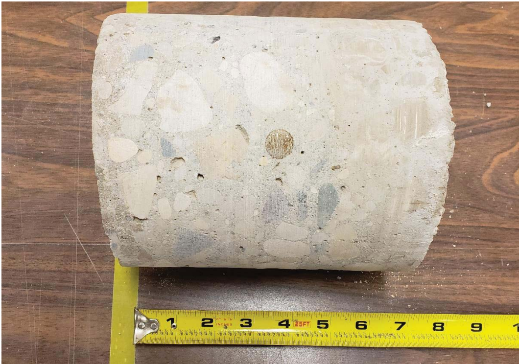
Figure 6 – PC-09 Inglewood Street
