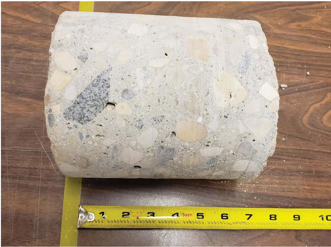
Figure 7 – PC-10 Inglewood Street
